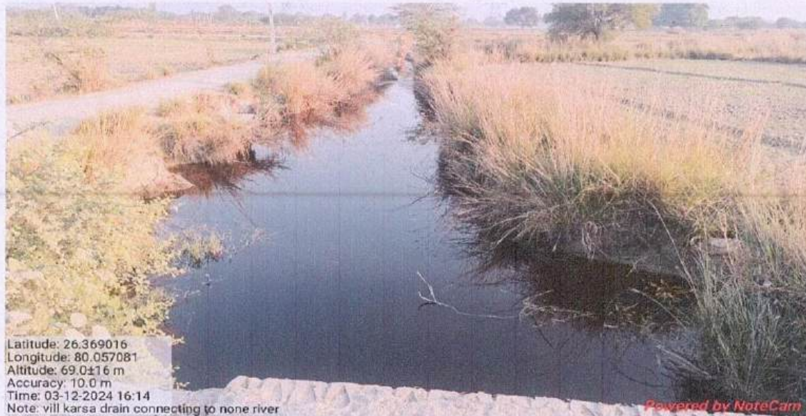
Patari Drain at Bilsarayan
